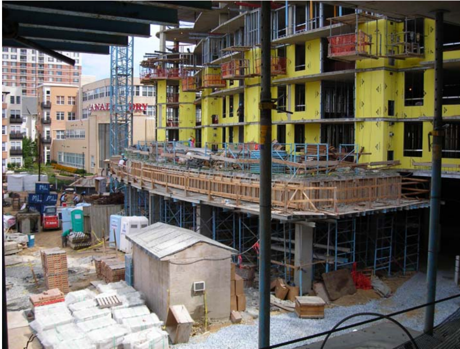
Photo 5: Partial view of lower floor construction on East-West Highway elevation (Southwest).
