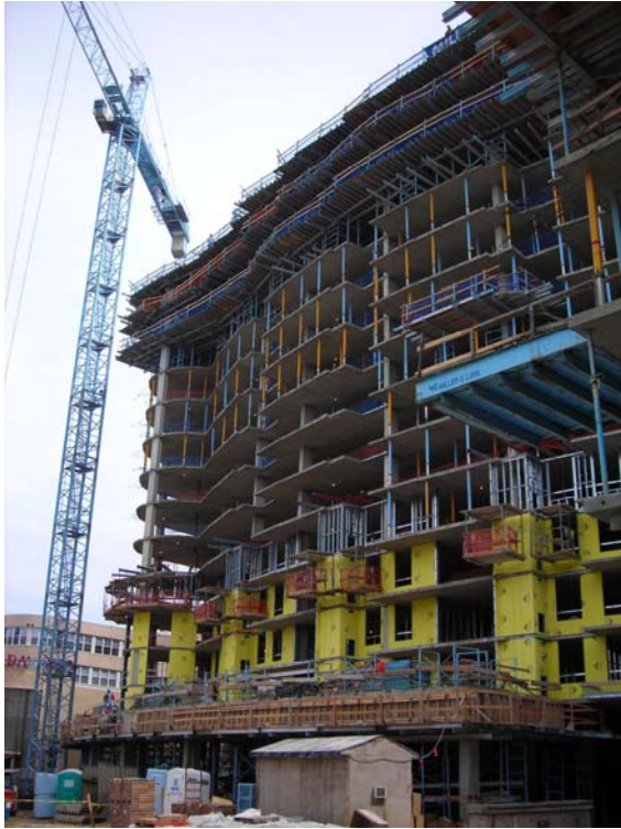
Photo 3: Partial view of the Southwest elevation.
