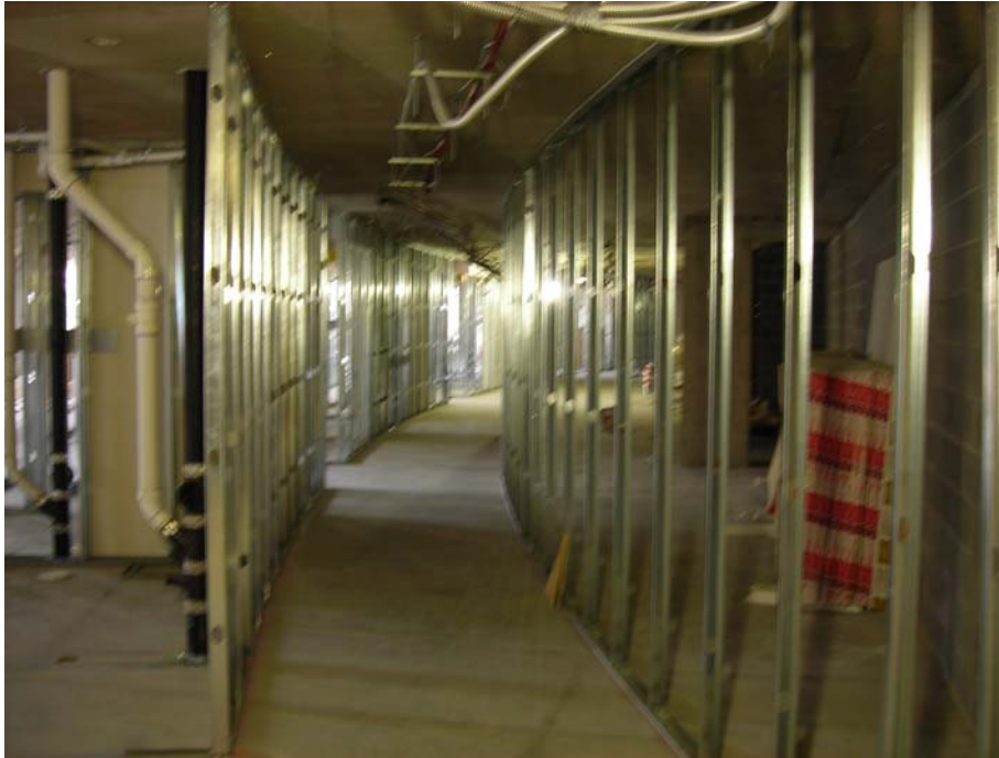
Photo 9: Interior view of a typical residential corridor.
