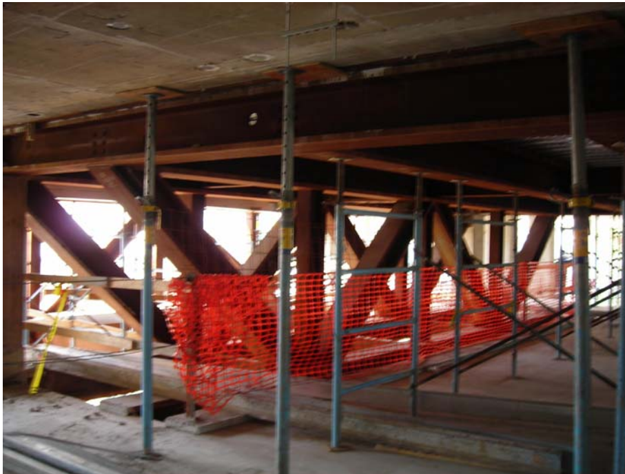
Photo 7: Interior view of pedestrian bridge steel structure.
