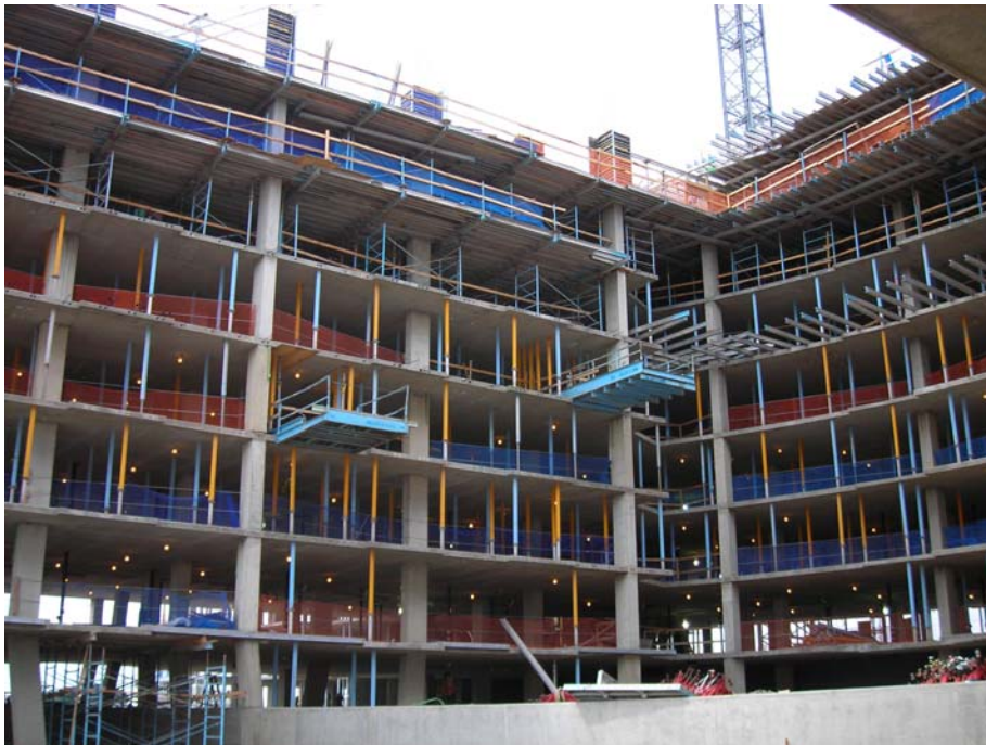
Photo 2: Partial view of courtyard from the top level of the parking garage.
